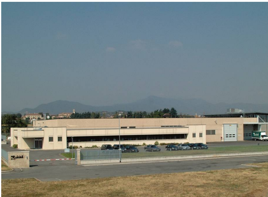
Photo 3: Factory in Cazzago San Martino
